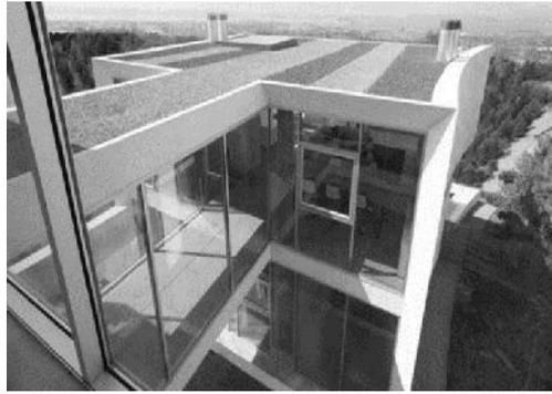
**Gambar 4.40 Atap Dak Beton**
