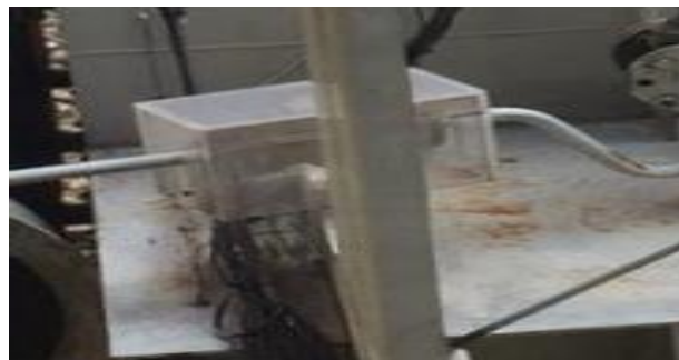
Gambar 2.16 Relay Bucholz Gi Mabar (Sumber :Gardu induk mabar,2019)
