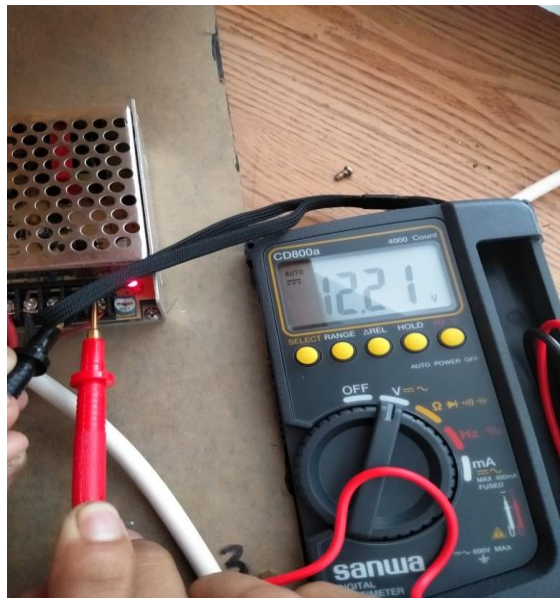
Gambar 4.1 Pengujian Power Supply
