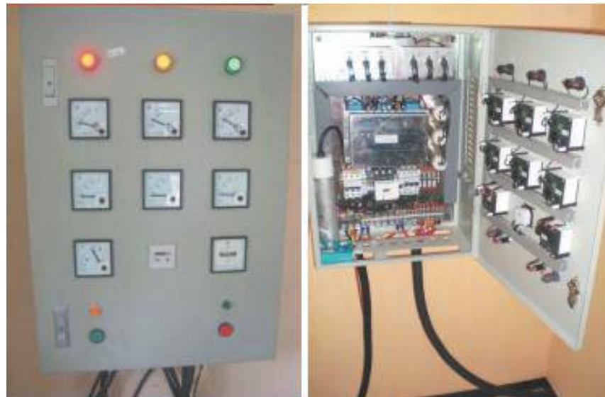
Gambar 2.8 Electronic Load Control (ELC)
